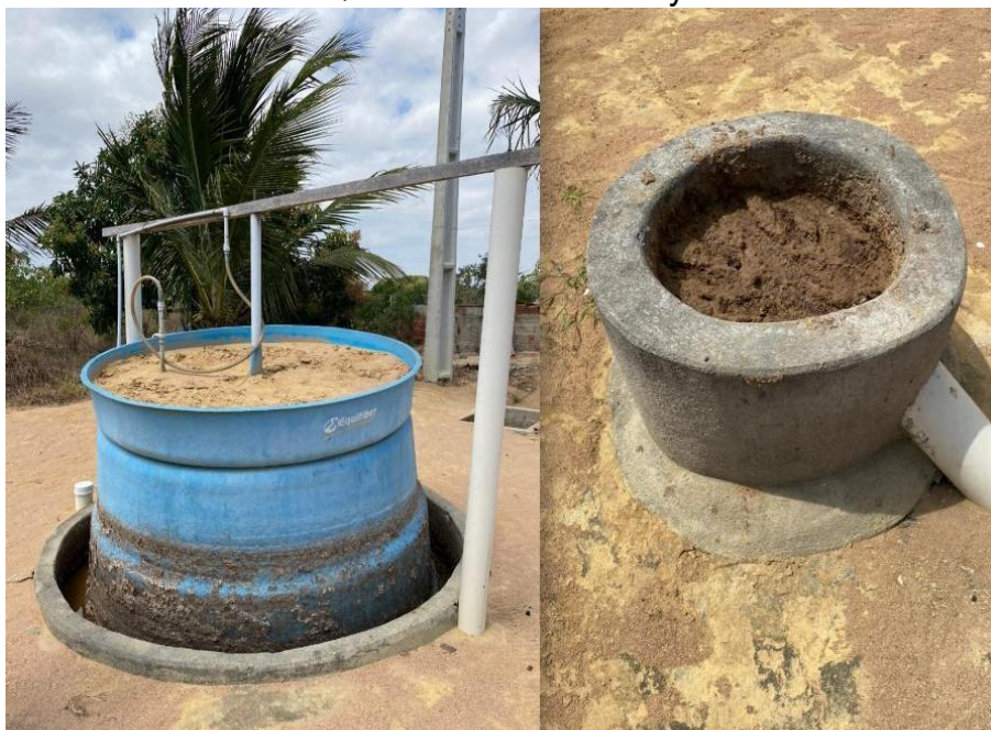
Figure 03 – Biodigester Installed by the Diocesan Caritas of Caicó in the Macambira Quilombola Community
