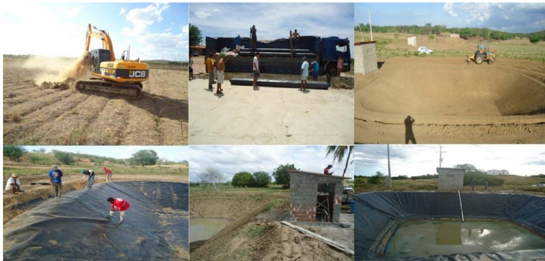
Figure 02 – Excavation, lining and construction process of reservoirs and pump houses
